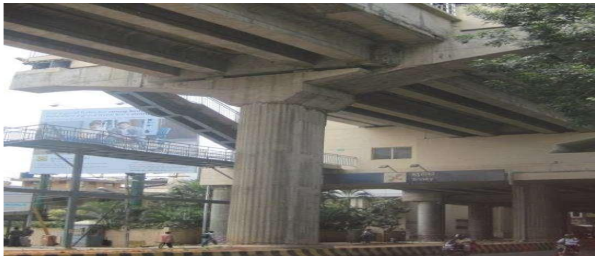
(a) Typical pier
